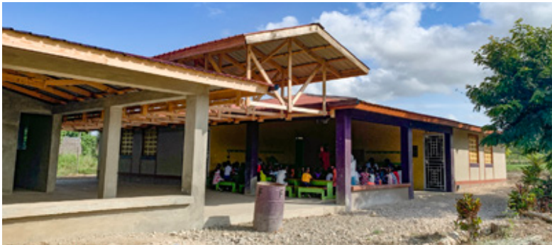
Front of the School of Light with new additional classrooms
