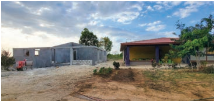
Construction of the new school building on our Sylvain campus
