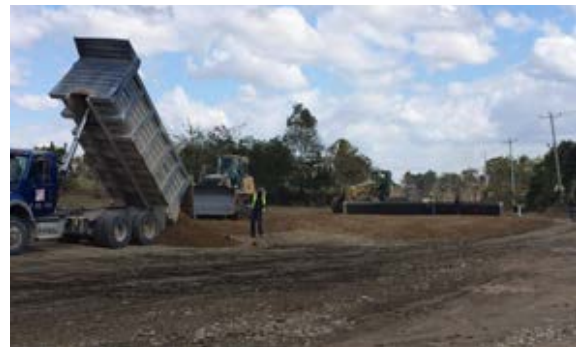
Government road work is continuing, with construction reaching Pignon
