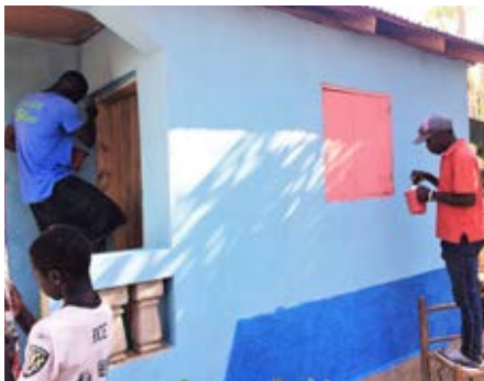
Haitian work crew painting a recently built house
